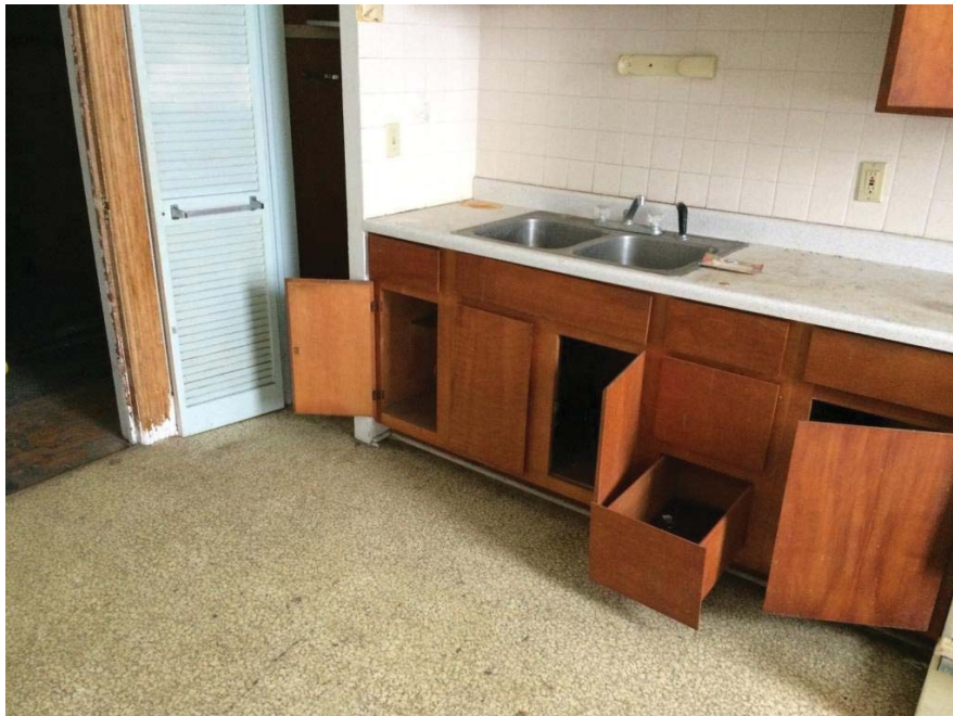
Linoleum, Sink Insulation & Wall Tile Adhesive – Kitchen 203
