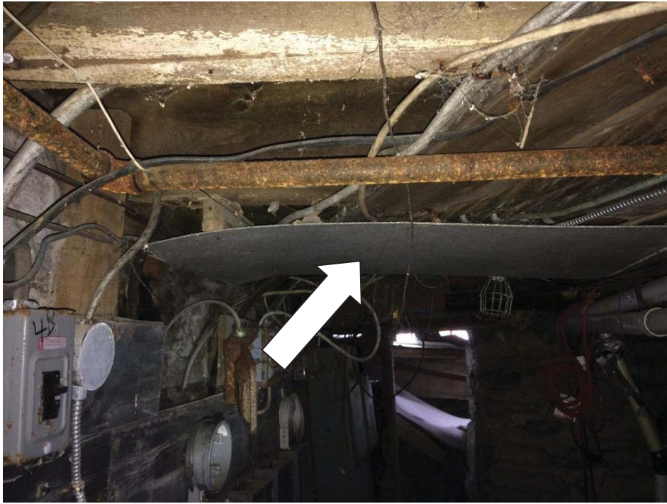
Cement Board – Basement Ceiling
