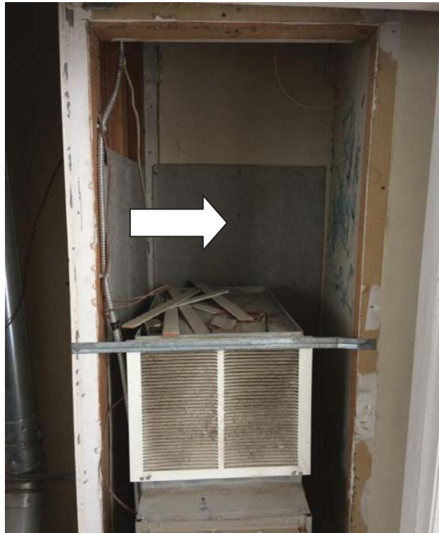
Cement Board – Room 200 Heater Closet
