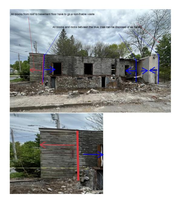
demolition with asbestos starts at vertical red line - lines are on the building right of red vertical line can be disposed of as hard fill.
