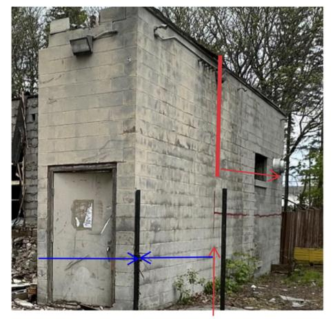
demolition with asbestos starts at vertical red line - lines are on the building left of vertical red line can be disposed of as hard fill.
