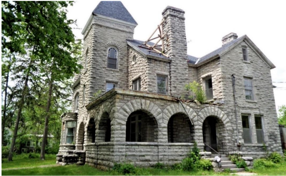
Fig.6: South East Facade
