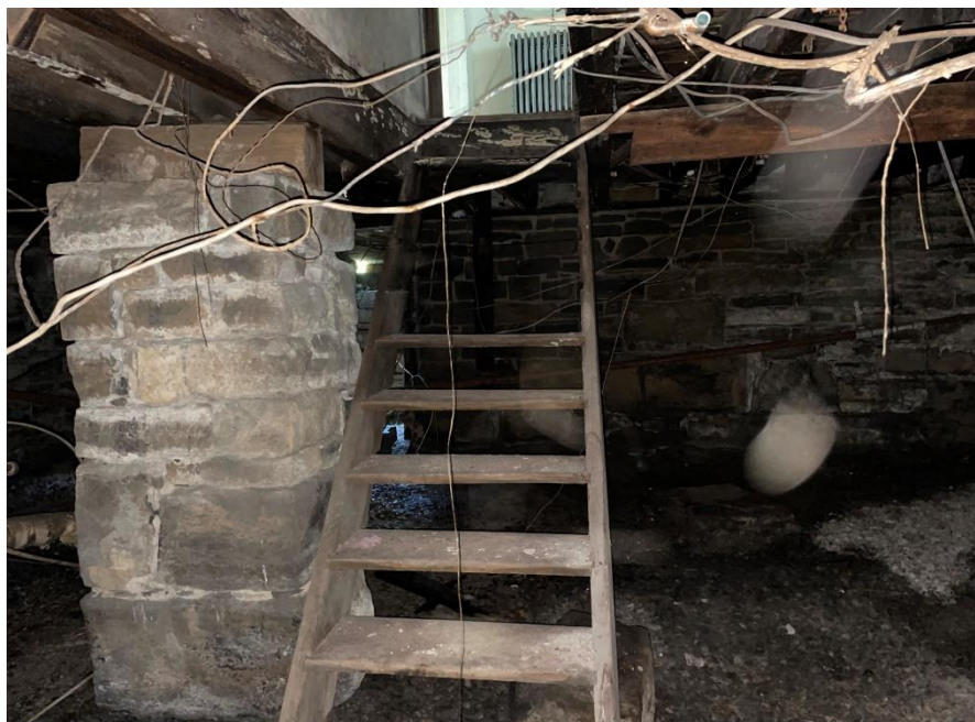
Fig.48: Stairs to the Basement
