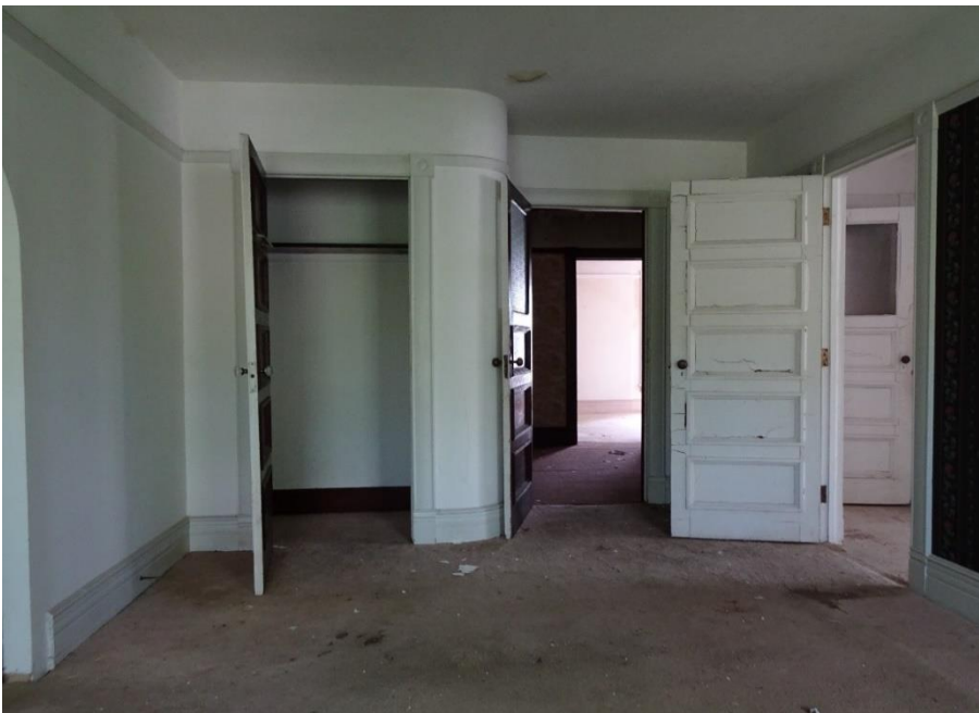
Fig.27: Second Floor, Looking West, Room 201
