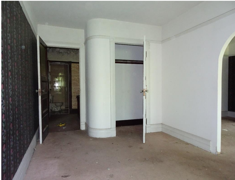
Fig.36: Second Floor, Room 212
