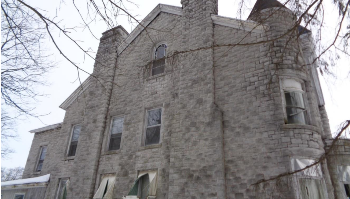
Fig.8: West Facade Windows
