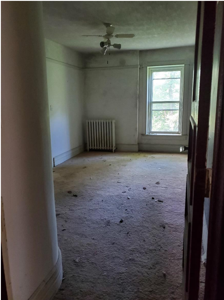
Fig.28: Second Floor, (Room 210)
