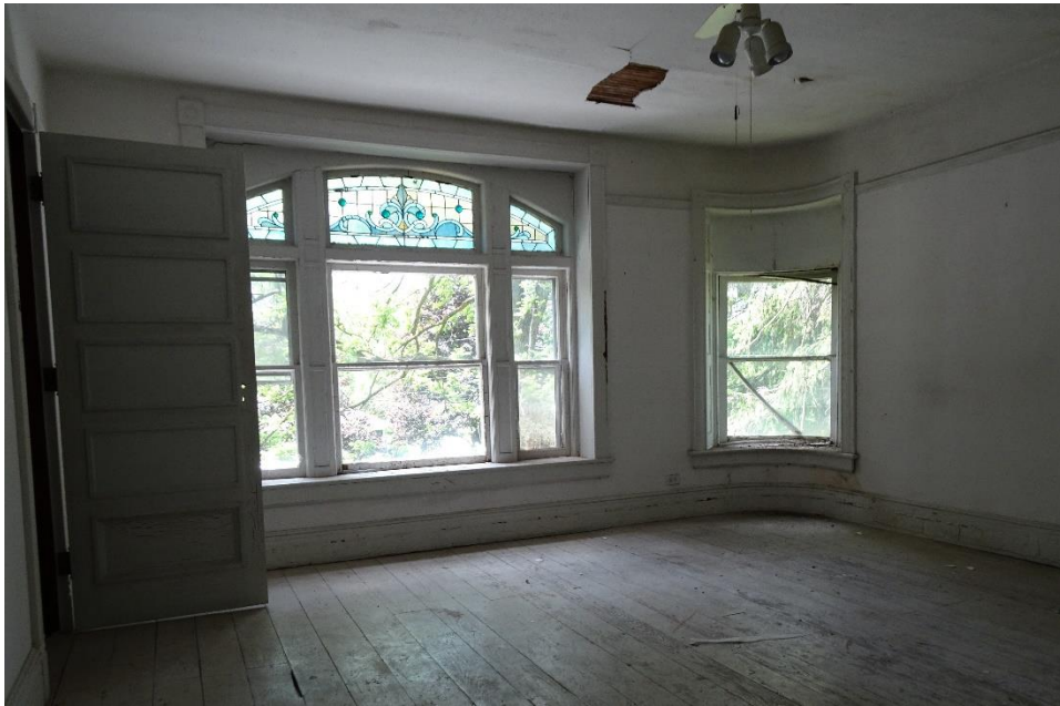
Fig.38: Second Floor, Room 214
