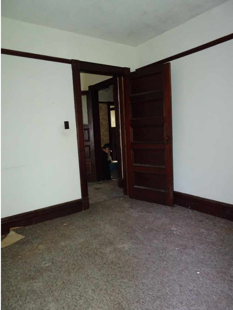
Fig.30: Second Floor, Looking North West, Room 208
