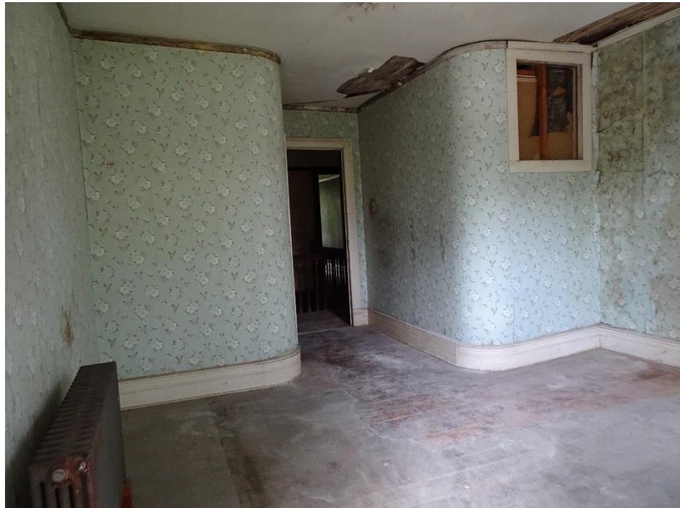
Fig.41: Second Floor, Room 203
