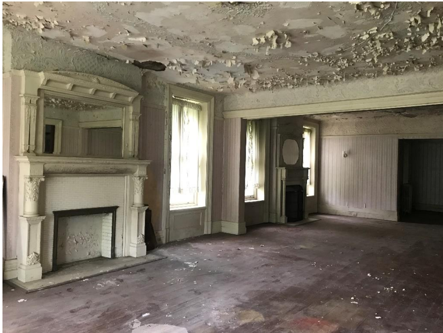
Fig.20: First Floor, Looking North, Room 110
