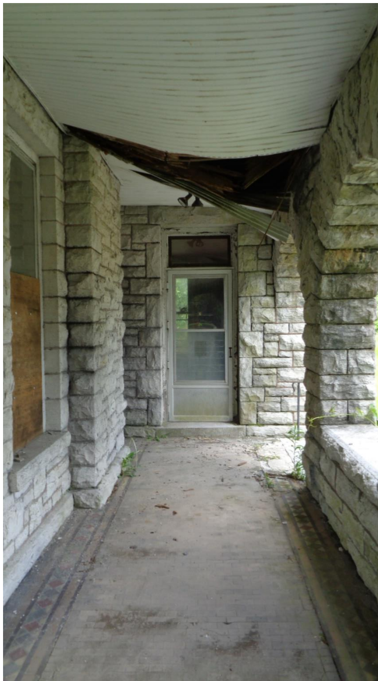
Fig.10: East Porch Roof
