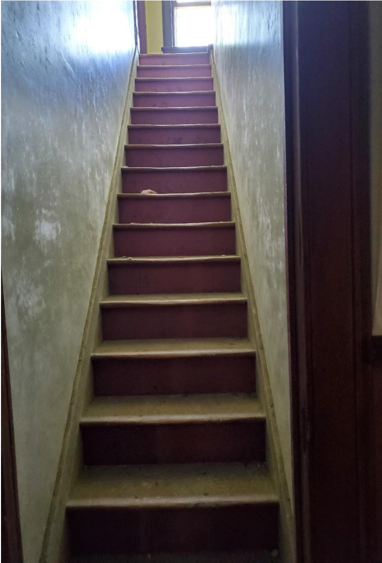
Fig.24: Stairs to the Second Floor
