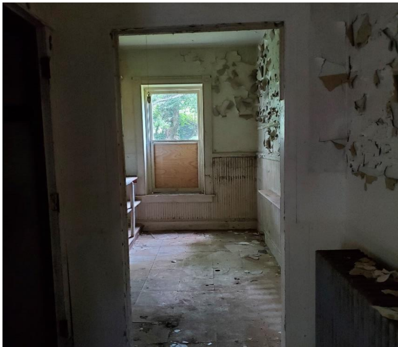
Fig.23: Storage Room, Room 108
