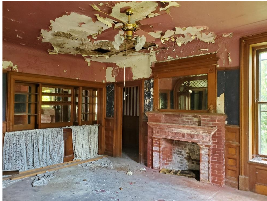
Fig.16: First Floor, looking North West, Room 103
