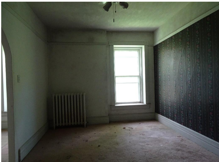
Fig.37: Second Floor Room 212
