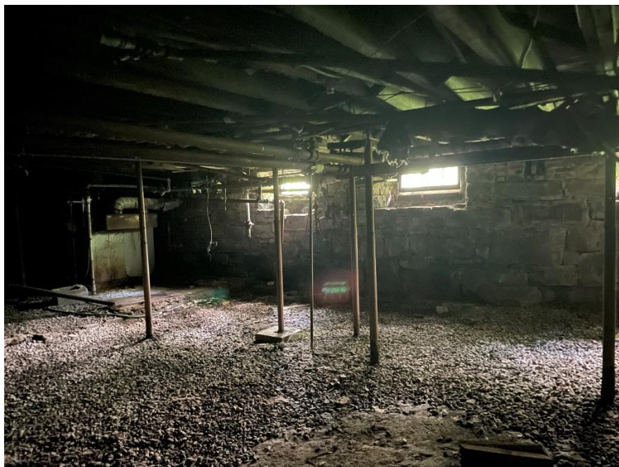
Fig.49: Basement Roof Condition
