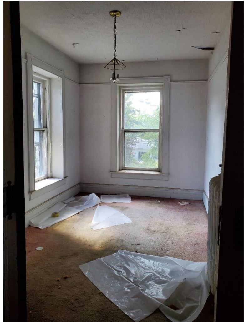
Fig.29: Second Floor, (Room 216)
