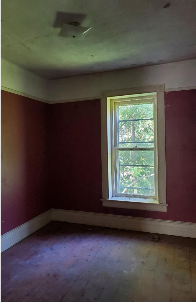
Fig.34: Second Floor, Looking West, Room 209
