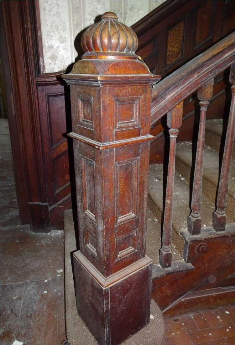
Fig.14: Staircase Hand Rail Detail
