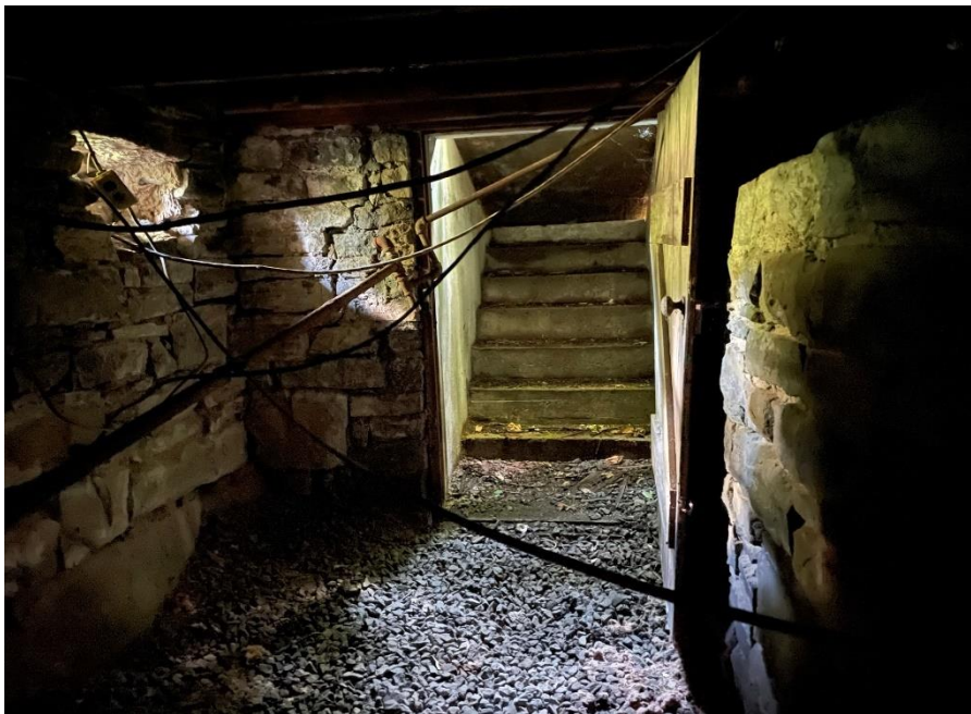
Fig.51: Back Door on the Basement
