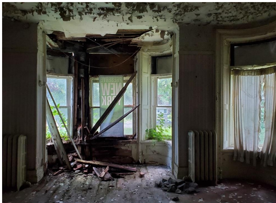
Fig.19: South Elevation Window, Room 110
